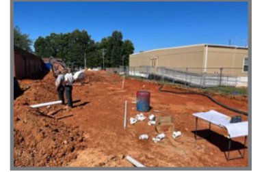
Footings & Underground Plumbing
