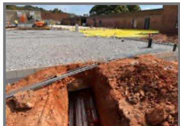
Final Underground plumbing, electrical and slab prep
