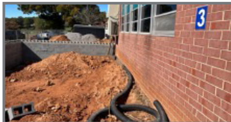
Final Underground plumbing, electrical and slab prep
