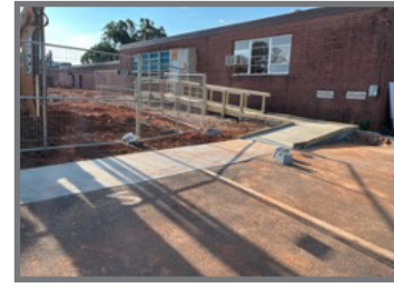
Installation of New Walks/Ramps
