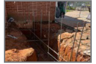
Footings & Underground Plumbing
