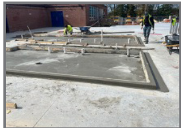
Group Bathroom Slab Prep
