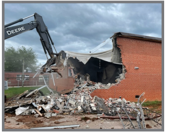
Demo of 1950 Building - July
