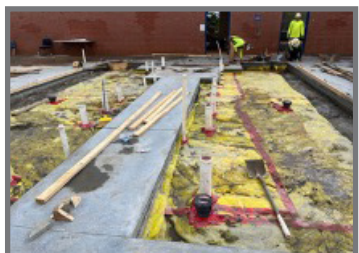
Group Bathroom Slab Prep
