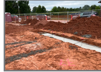
Footings & Underground Plumbing
