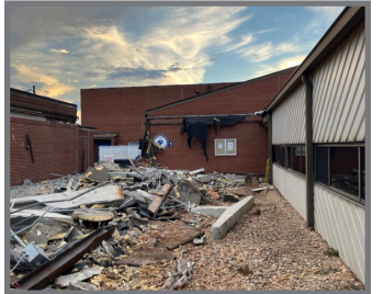
Demo of 1950 Covered Walkways - July
