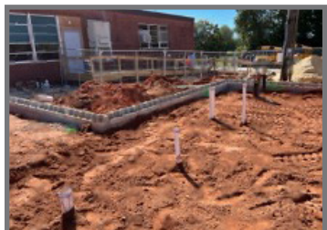
Final Underground plumbing, electrical and slab prep
