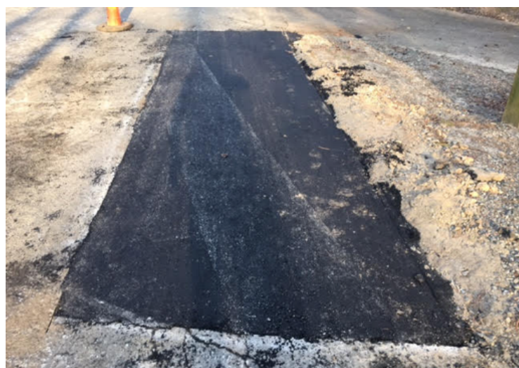
Properly repaired pothole
