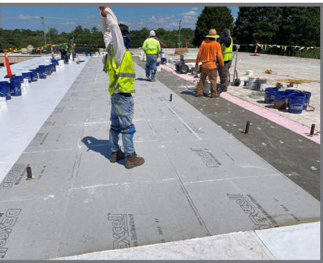
New re-cover insulation and cover-board being installed over the exist-ing insulation system
