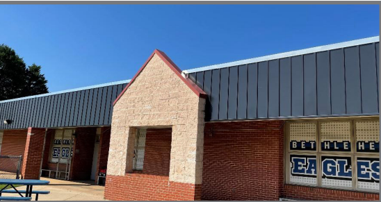
New parapet wall at old mansard
