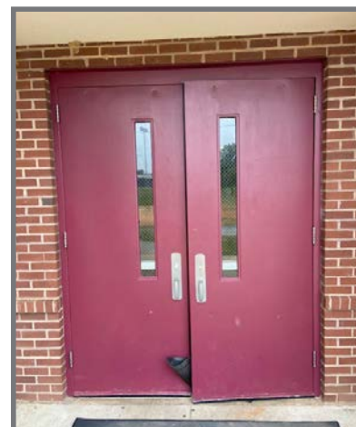
Before - Hall Exit
