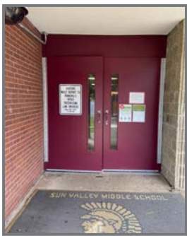
Before - Hall Exit
