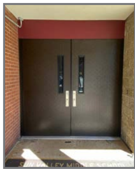
After - Hall Exit
