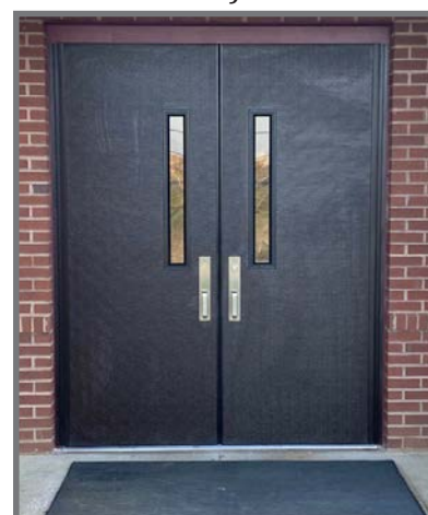
After - Hall Exit
